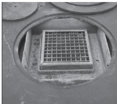
Figure 9 Hotplate Removed Showing Internal Flue Way
