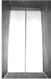
2. Note that the two back bricks are wider than the side bricks. Do not confuse them.
